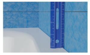
Place the tape with the top edge along the previously made marks. The adhesive strip on the backside ensures an easy fixation of the tape.
